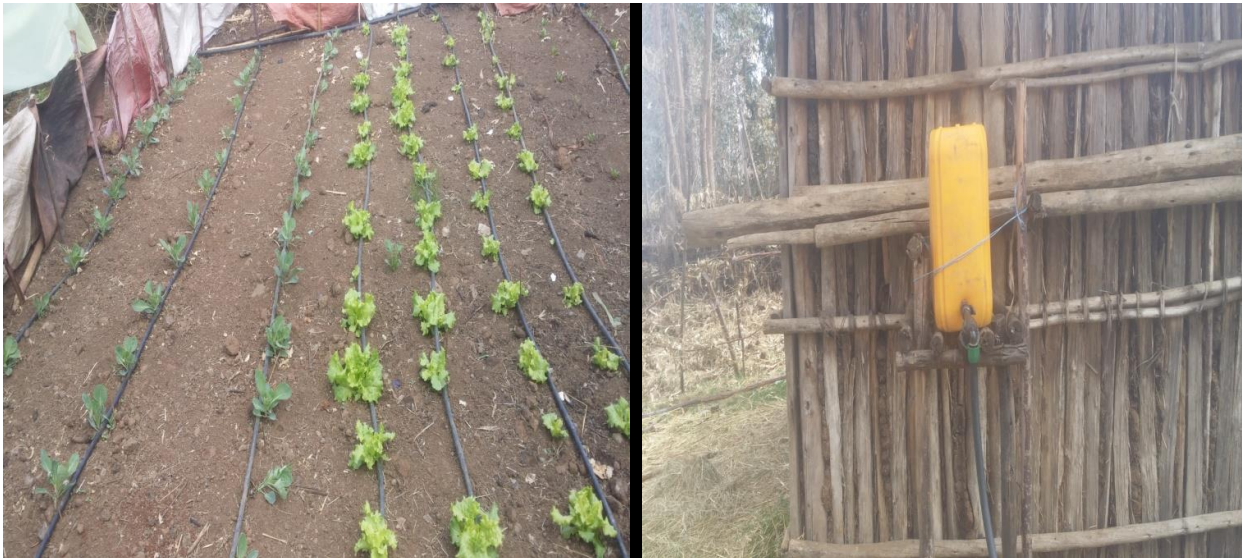
Fig. 2: Photos of drip line installation and rope and washer pump.
